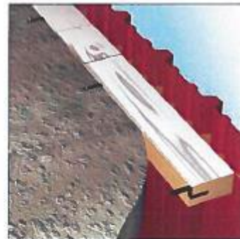
Close up of Spanatherm support bracket
